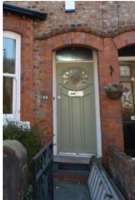
Though tasteful and in good condition, this Inter-War style door is not of the appropriate period for the house
