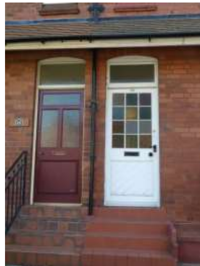
Style seven: An original door to No.17 Norman Road (right) and a replacement door to No.15 Norman Road (left)
