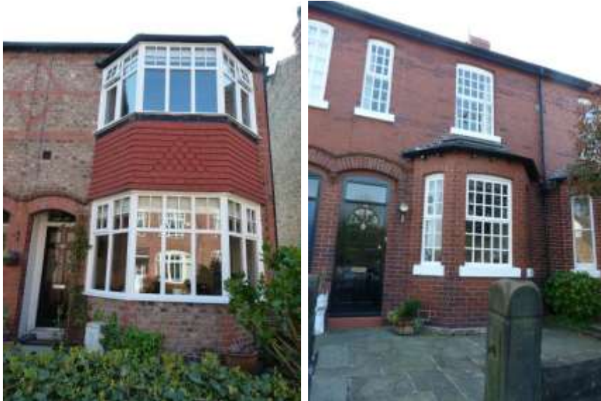
Inappropriate double height bay window at No. 42 Weldon Road
