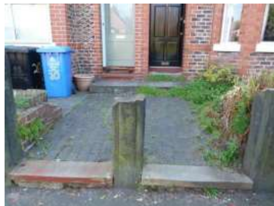
Original diamond pattern textured paving to Nos. 18 and 20 Weldon Road, together with damaged original stone gateposts
