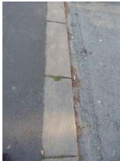
Historic kerb stones on Weldon Road
