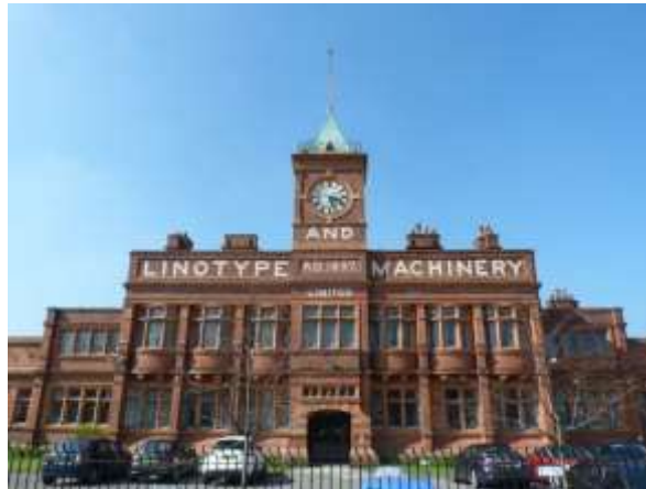
The main elevation of the Linotype Works
