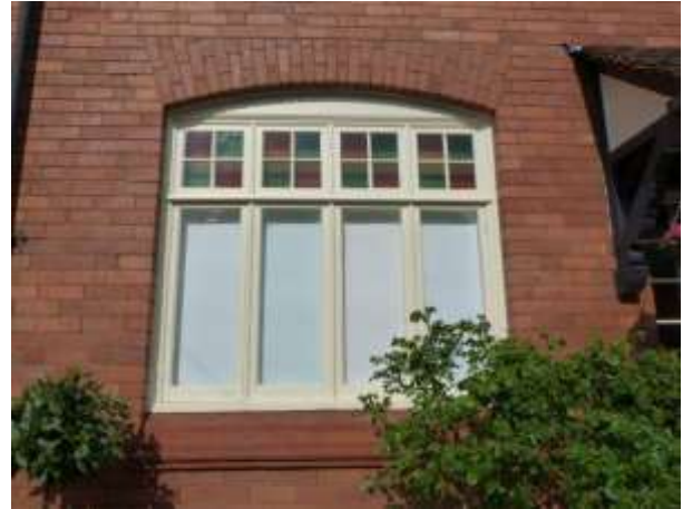
An original window at No. 9 Weldon Road
