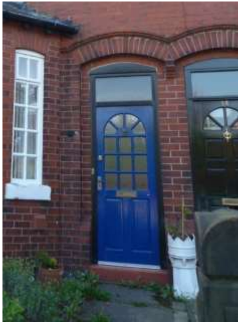
Inappropriate Georgian style doors to Nos. 14 and 16 Weldon Road, though both have their original fanlights surviving
