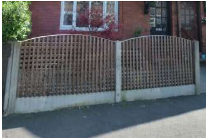
An inappropriate fence at No. 47 Norman Road which is too tall and its more solid character reduces the sense of openness to gardens in the conservation area
