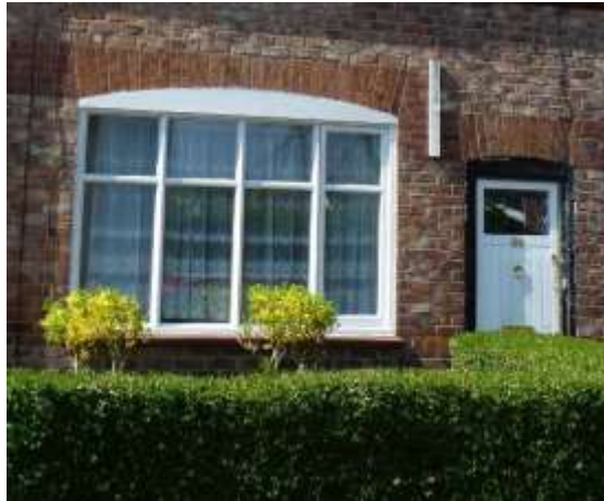
Detail of original window (note side hung casement to the side of the window nearest the door) and door at No. 66 Lock Road
