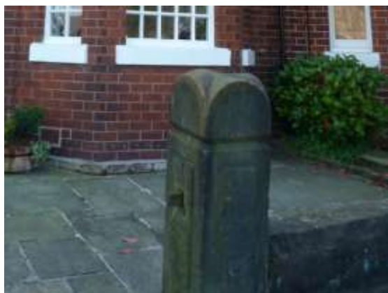
Original stone gatepost and garden wall at No. 14 Weldon Road
