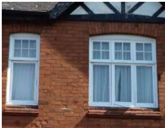
Style Six: First floor windows to No. 59 Lock Road showing side hung casements to lower panes
