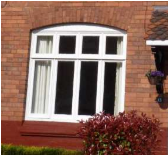
Ground floor window to No. 13 which lacks the groups of four small upper panes
