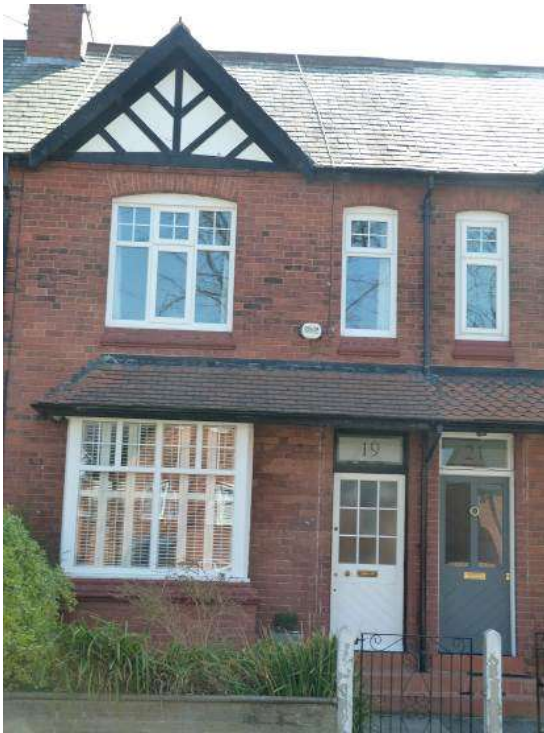
A typical style six house at No. 19 Norman Road
