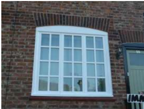
Timber framed window at No. 55 Lawrence Road
