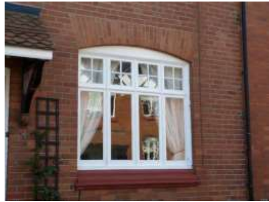
Style Six: Original window at No. 3 Pollen Road, though this example has lost its coloured glass
