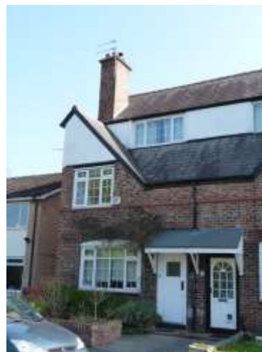
Porches added to Nos. 79 and 81 Lawrence Road
