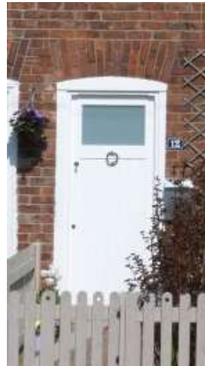
uPVC example of a door which follows the design of the original doors, No. 12 Bemrose Avenue
