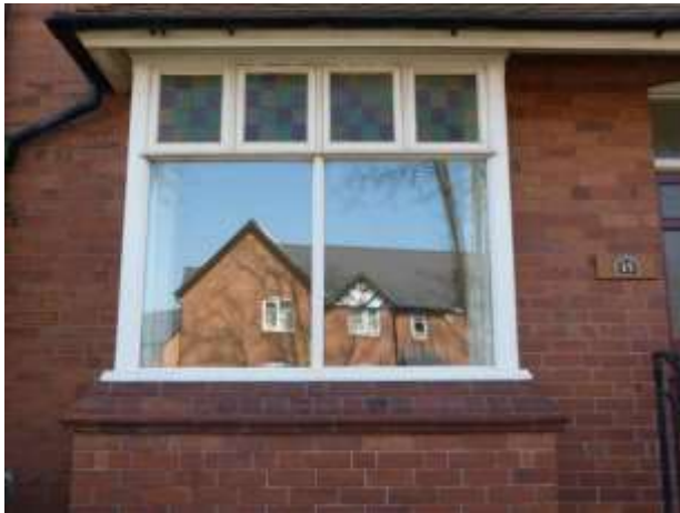
Style Seven: Original window frame to No. 15 Norman Road, though with possible replacement coloured glass panes
