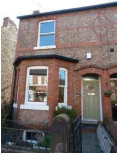
uPVC sash windows at No.44 Weldon Road
