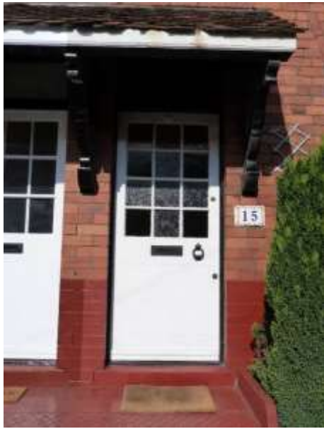
Original door to No. 15. Some of the coloured glazed panes have been replaced with textured glass
