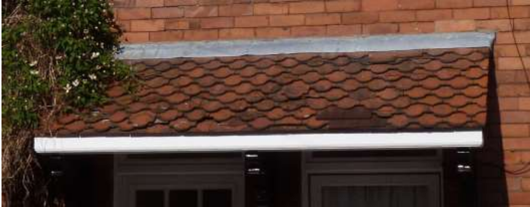
Detail of a porch. Some of the scalloped tiles have been replaced with straight edged ones, disrupting the pattern
