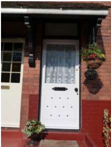
Adapted original door to No. 11, with a large pane of glass to the upper half and studding to the lower half
