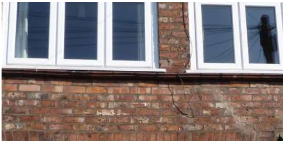
Moulded brick string course below the first floor windows
