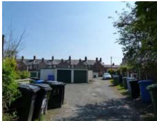
20 th century garages behind Place Road, Weldon Road and Lawrence Road
