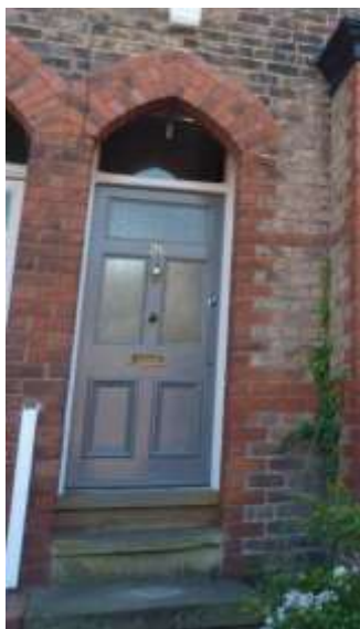
Original door at No. 26 Weldon Road
