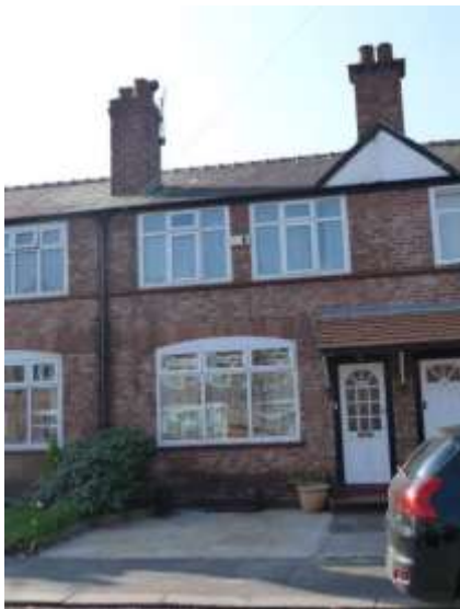
A front garden which has been paved over at No. 23 Place Road
