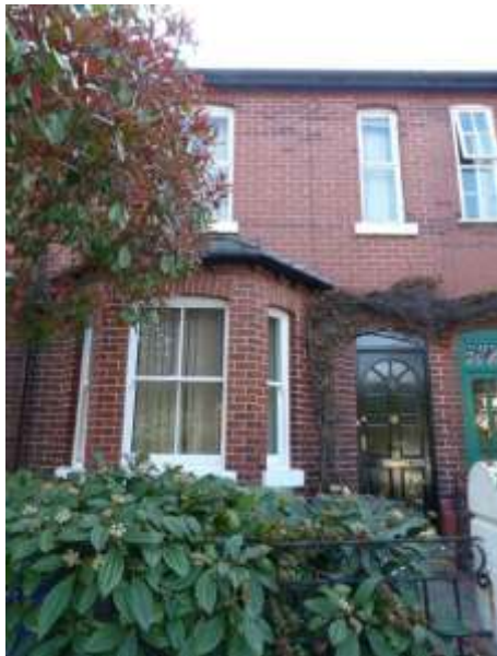
A typical style two house at No.12 Weldon Road. This example has original windows but a replacement door
