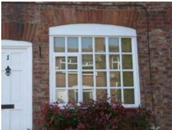
Timber framed window at No. 1 Place Road
