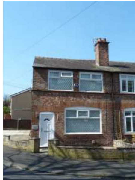
Inappropriate faux-leaded windows at No. 72 Lock Road, with frames that do not match the original composition
