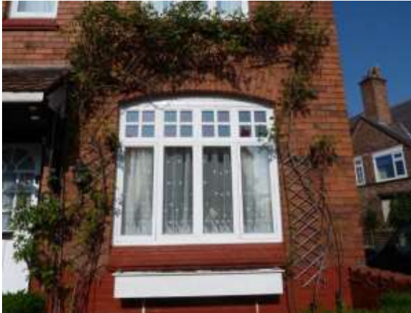
An original window at No. 19 Weldon Road
