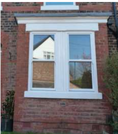
uPVC sash windows to No.22 Weldon Road in an appropriate design mirroring the original timber versions
