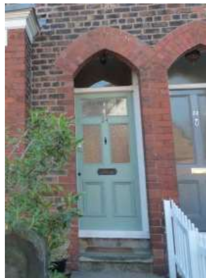
Original door at No. 24 Weldon Road
